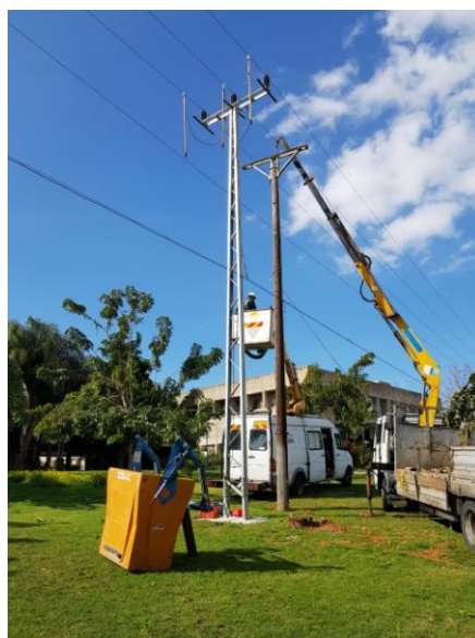
Fig. 1: The new metal pole next to the old wooden one
