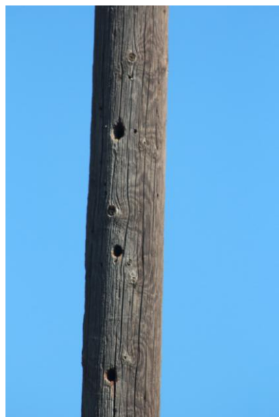
Fig. 2: Holes in the electricity pole made by the Syrian woodpecker (Photo Henk Mienis)
